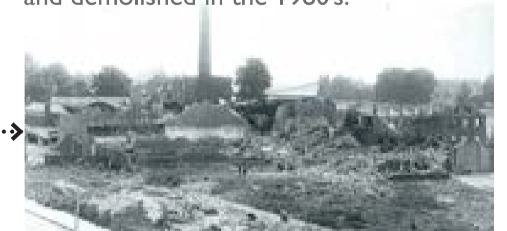
Buildings destroyed by a VI flying bomb on 24 July 1944. The area is now covered by Furnivall Gardens.
