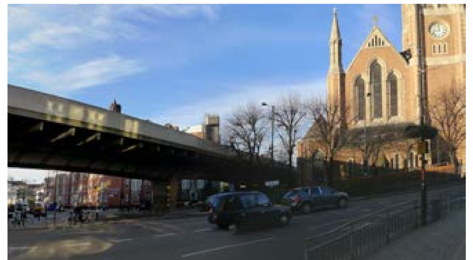
Current view of the flyover in the context of St Paul's Church
